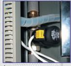
Inbuilt electrothermic valve controls the outlet or room air temperature.
